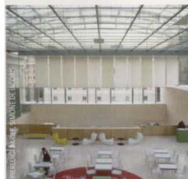
8 RECONSTRUCTION OF PIACENTINI'S GREENHOUSE (2007) Architect: ABDR Architetti Associati Address: Via Milano/Via Piacenza
