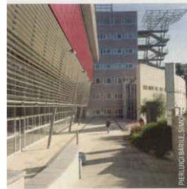
12 UNIVERSITY COMPLEX (2006) Architect: spsk Address: Via Silvio D'Amico 77
