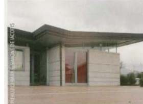
18 CIAMPINO MULTIFUNCTIONAL CENTRE (2003) Architect: n:studio Address: Via Stabilia 18
