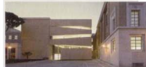
10 NEW LATERAN UNIVERSITY LIBRARY (2006) Architect: Jeremy King, Riccardo Roselli Address: Piazza S. Giovanni in Laterano 4
